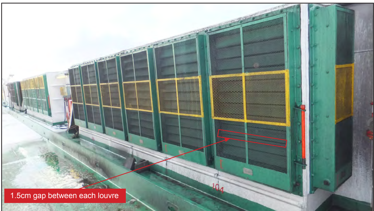
Figure 9: Main deck ventilation jalousie
