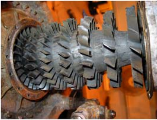
Figure 3 Compressor wheel with third stage bent blades
