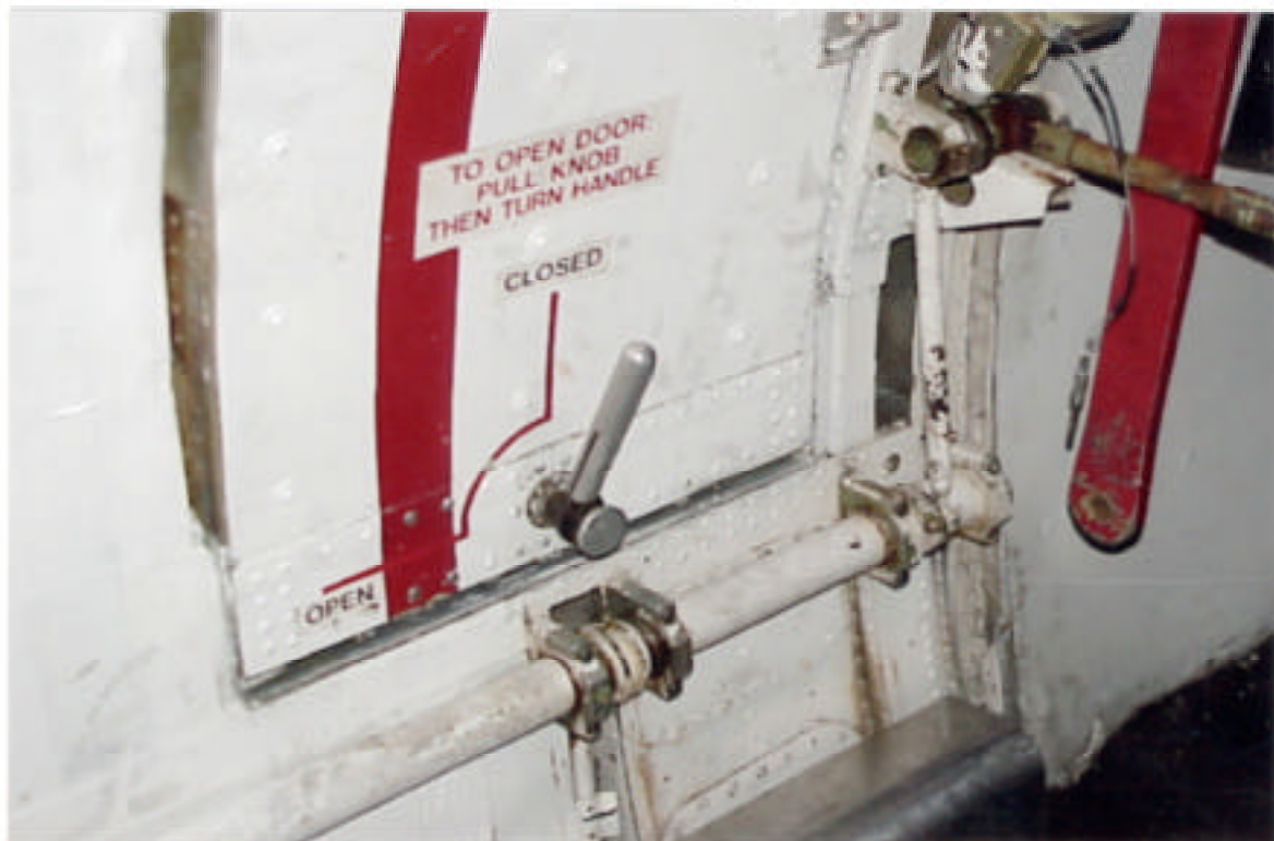
Photograph 4 Crew Emergency Exit Door fitted to the aircraft normally operated by the accident flight crew
