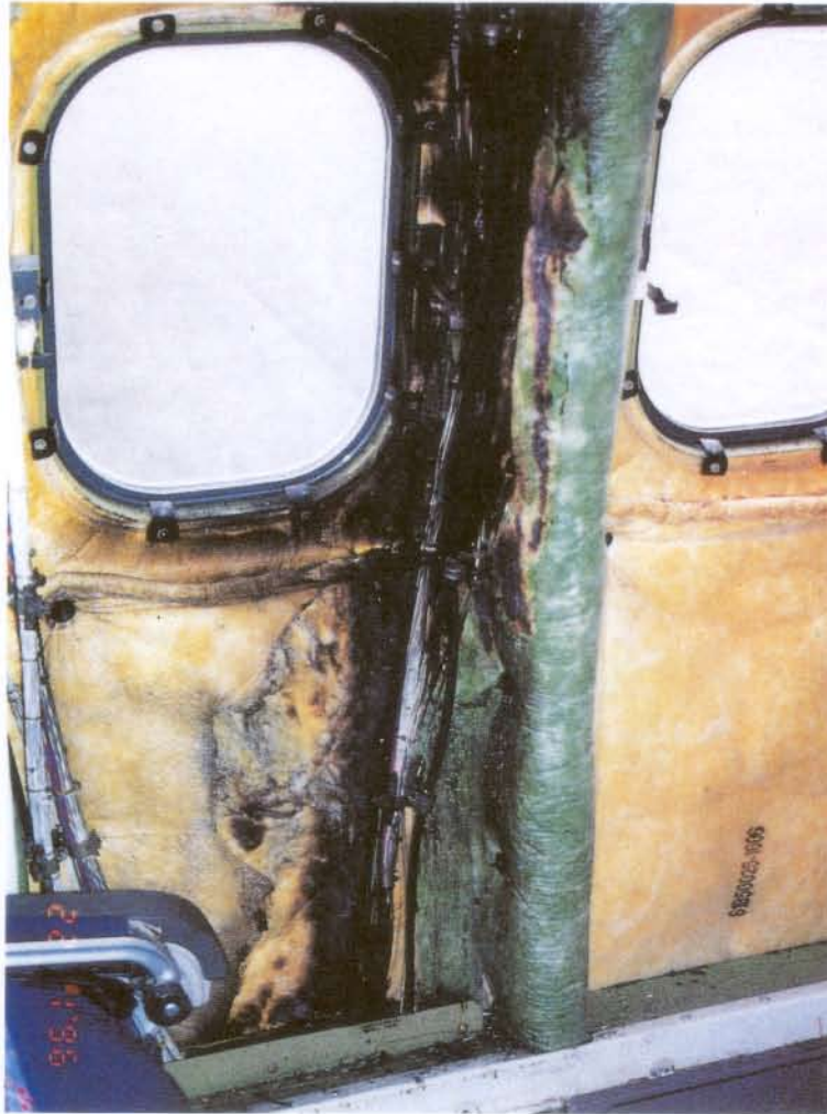
FIGURE 1. View of fire damaged area (trim panel removed)
