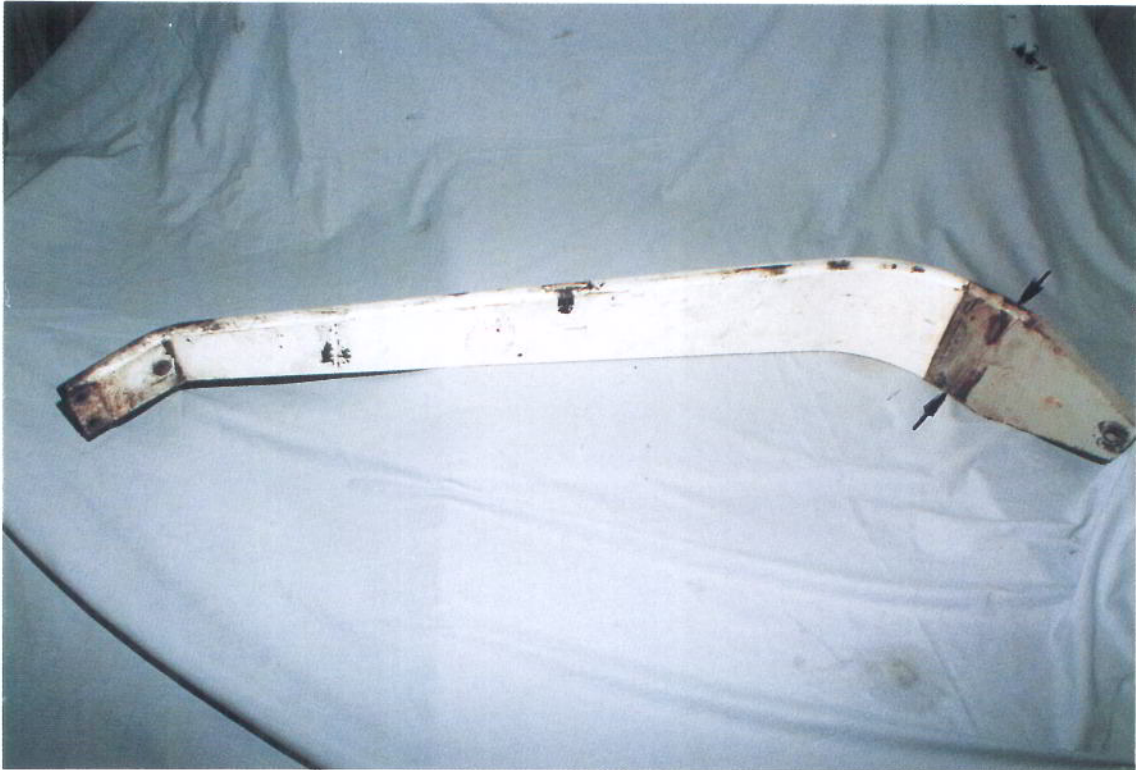
Fig 1: Left mainleg with position of fracture indicated by arrow
