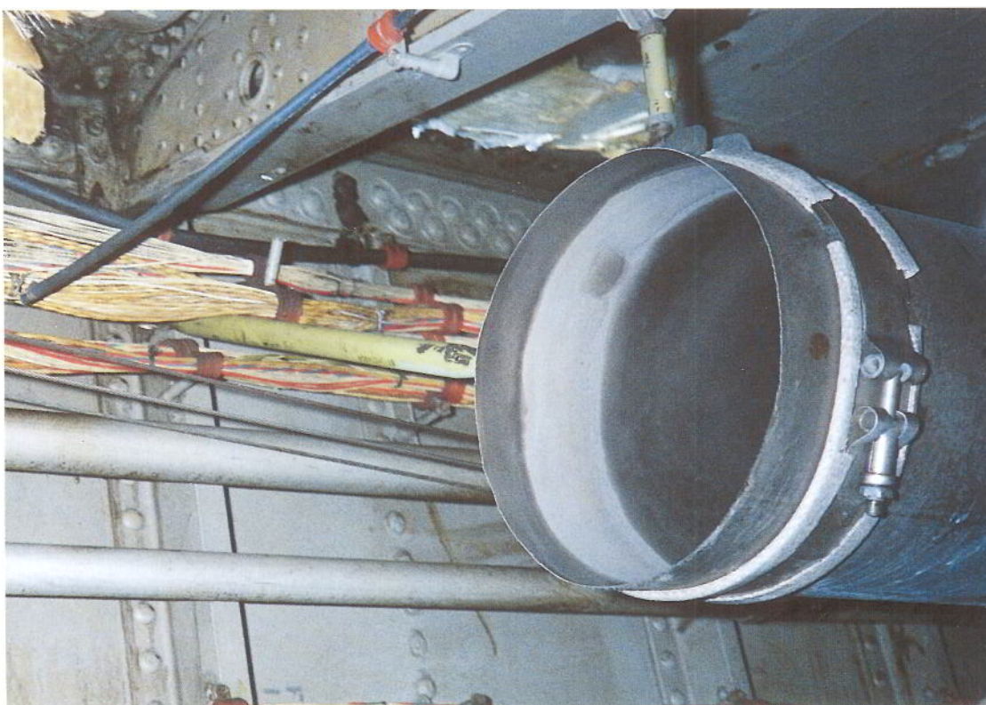
VIEW OF CIRCUMFERENTIAL FAILURE OF BLEED AIR DUCT AT WELD
