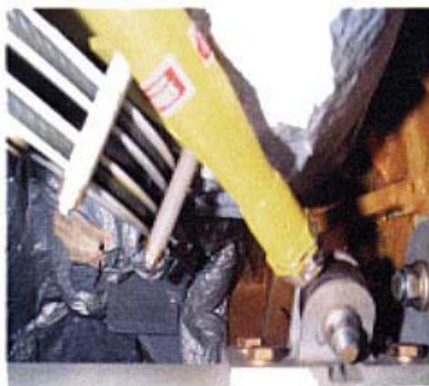
G-OINV - Photographs showing (above) dislodged insulation bag interfering with aileron cable and (below) with bag removed, the pressure bungs (note retaining button)
