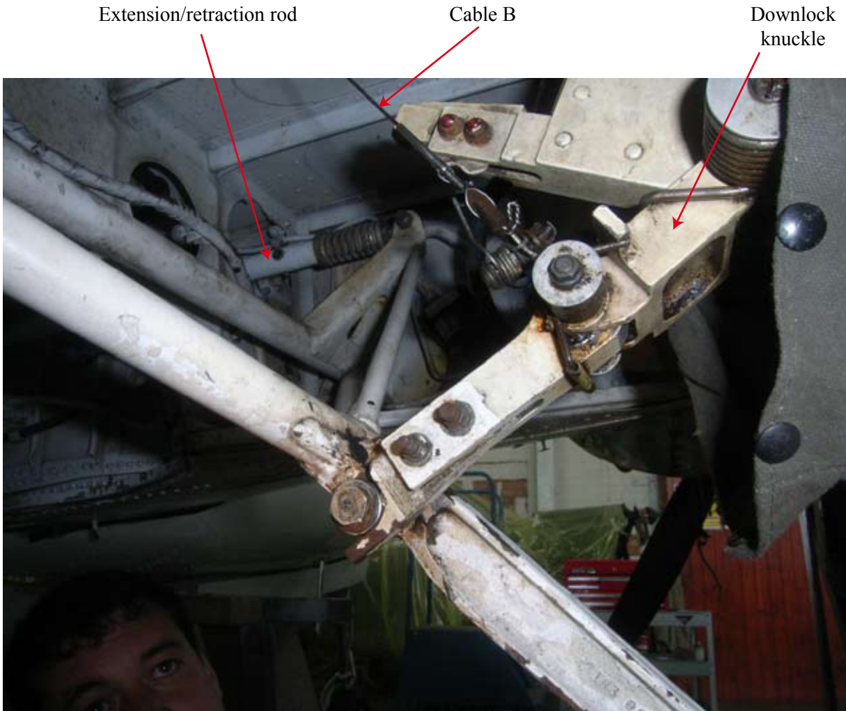
Figure 1 Gear down and locked
