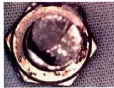
(Photo: H T Consultants) FIGURE 1b. Underside of fractured bolt head showing lack of damage to plating. Thrust face of associated nut showed similar lack of damage
