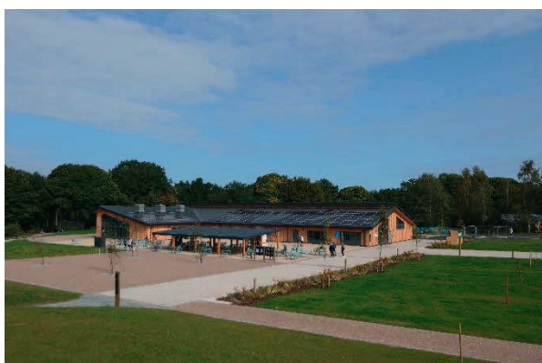
Figure 4: The completed Delamere site
