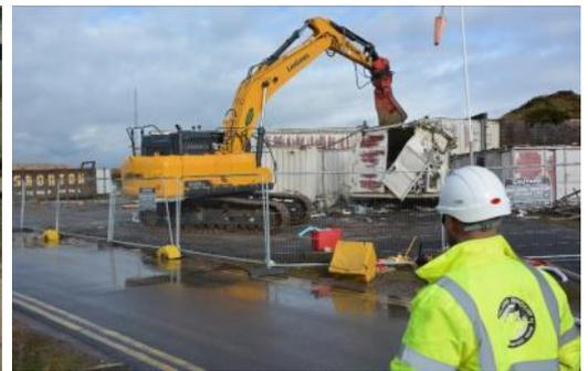
*Top: Personnel working in air-fed suits bag PCM in a Magazine Retrieval Facility (MRF), the blue buildings built on to the front of the magazines, as shown above in 2008, constructed in the 1990s, for containment of the contaminated material. Above right, Magazine 3's MRF is demolished and below, the magazines today, free from contamination and ready for demolition.*
