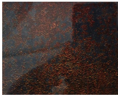
Figure 1-3 Rust Grade B
