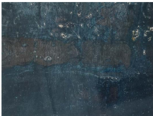
Figure 1-2 Rust Grade A
