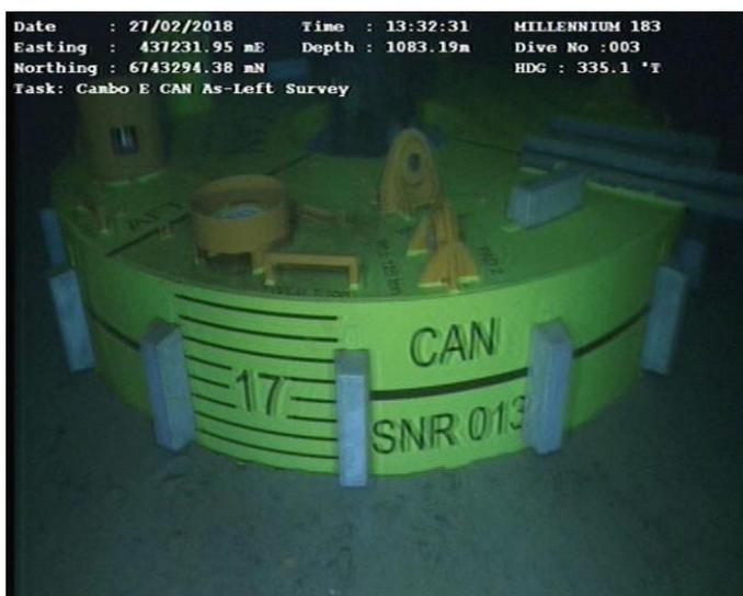
**Figure 3.5: CAN-ductor for the Previously Drilled Cambo 5Y Well Installed on the Seabed**
