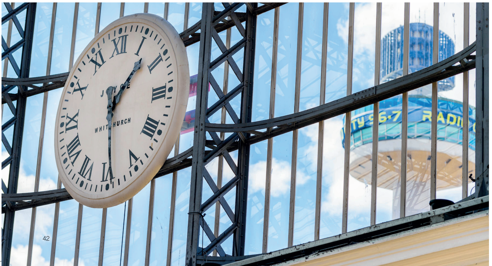
Liverpool Lime Street station
