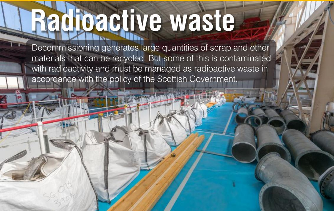
Low-active waste is compacted, cemented in containers and sent for disposal to a series of shallow engineered vaults adjacent to the site.
