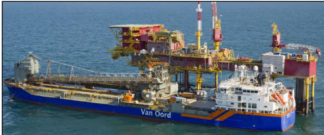
Figure B.5 – Rock Installation Vessel (Van Oord)
