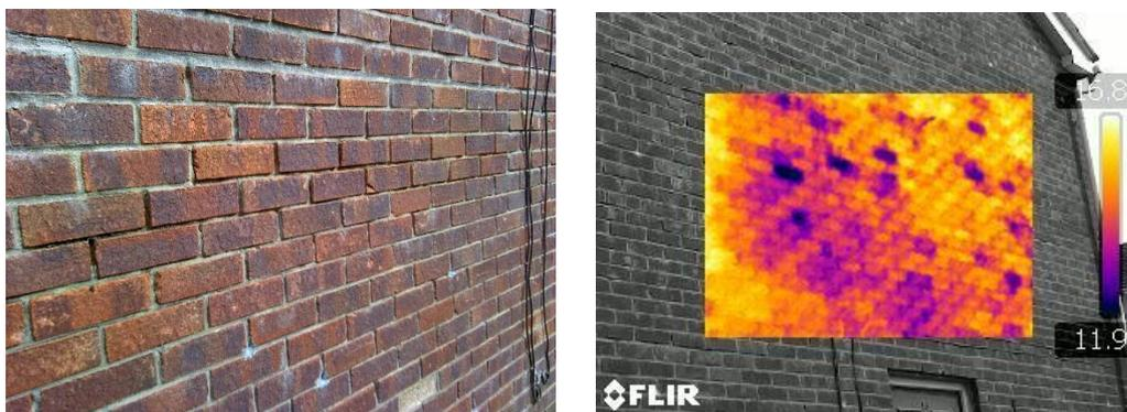
Figure 18: Examples of faults identified in facing brickwork: Left – Eroded mortar beds, Right – Saturated bricks caused by erosion or face damage
