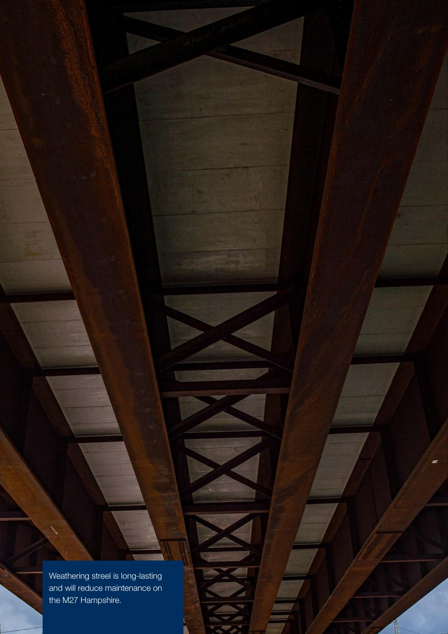
Weathering steel is long-lasting and will reduce maintenance on the M27 Hampshire.
