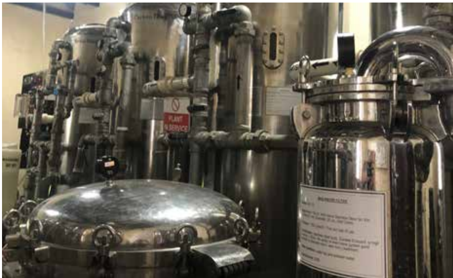
The filtration treatment process includes birm, carbon and resin filters © Crown
