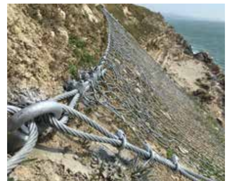
Freshly installed rock netting © Crown
