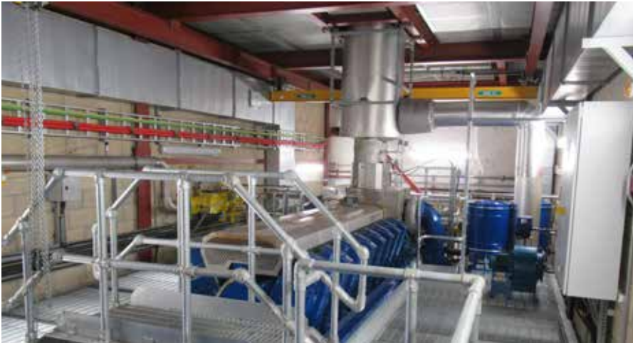
The Combined Heat and Power plant engine bay © Iain Greenlees
