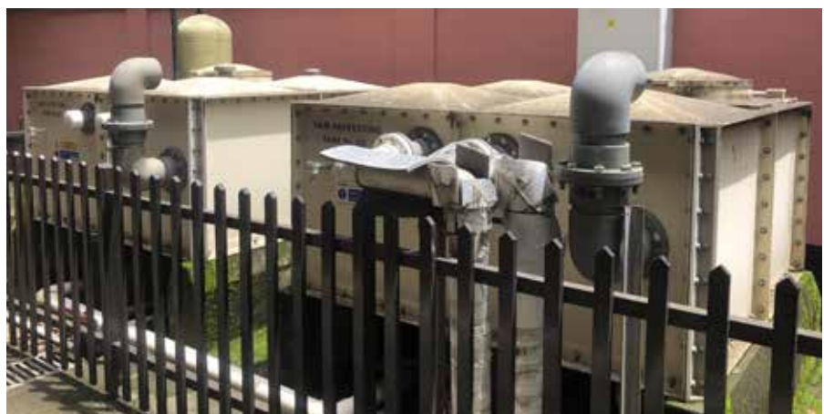
RWH storage tank and sand filter © Crown
