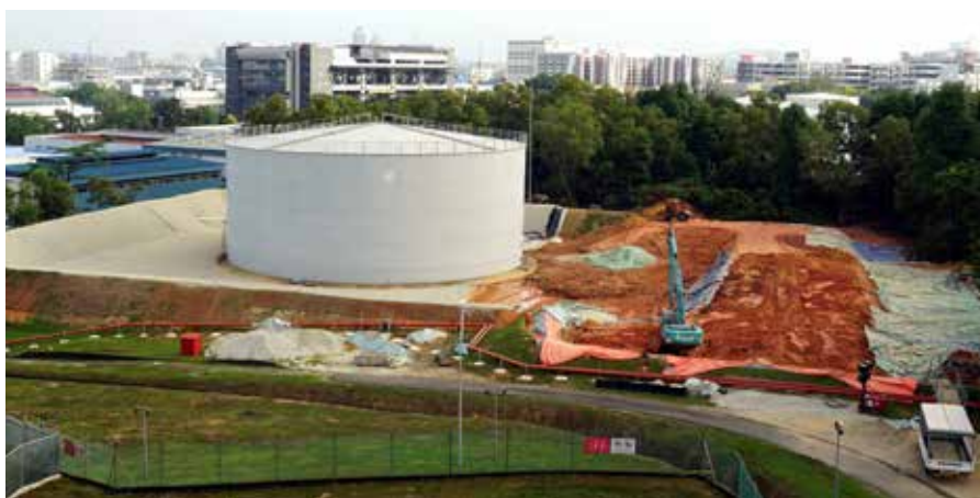
Bund clearance, forming and lining around Tank 12 © Andy Leishman
