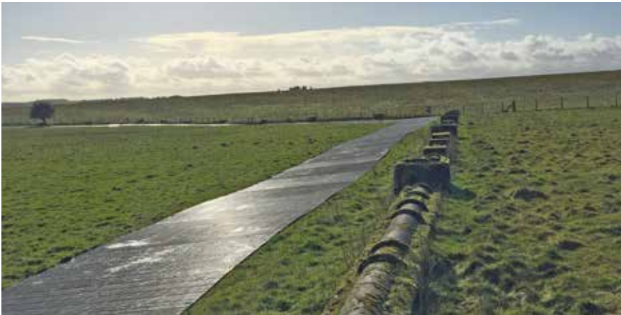
Existing soakaway pipe and support removal from the Stonehenge Cursus © Paul Chadwick
