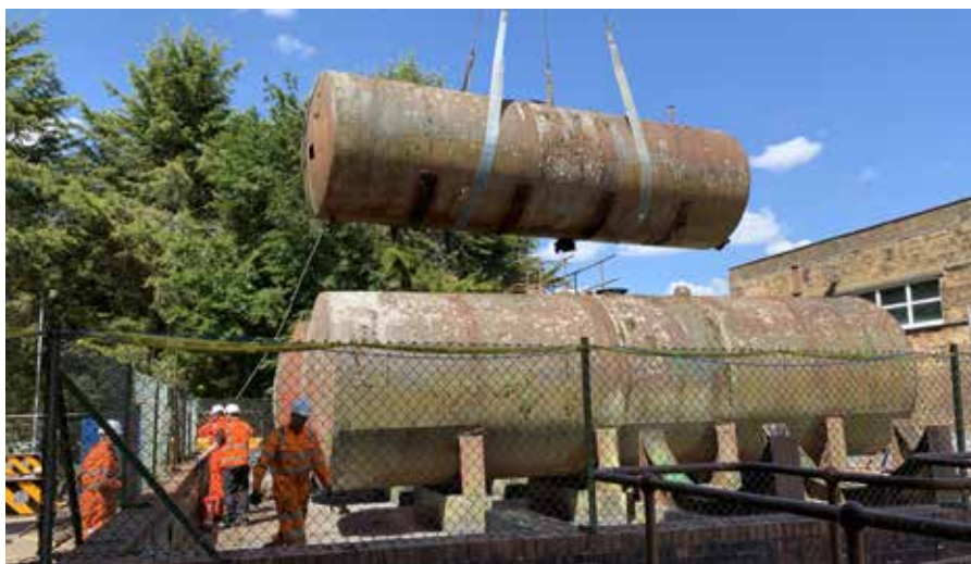
Removal of the tanks © LCM Environmental
