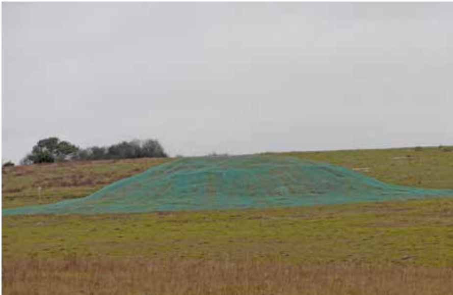
Completed chain mesh work on a tumuli © Dstl
