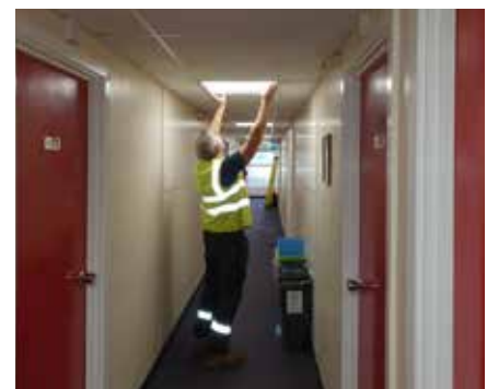
Installation of energy efficient LED lighting at HMS Collingwood © Mark Powell
