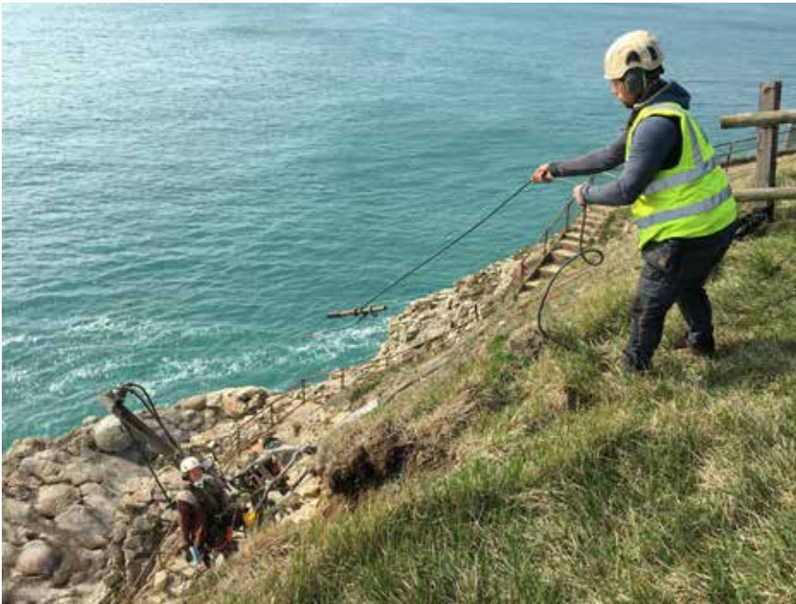
Vertical Technologies install new rock netting © Crown
