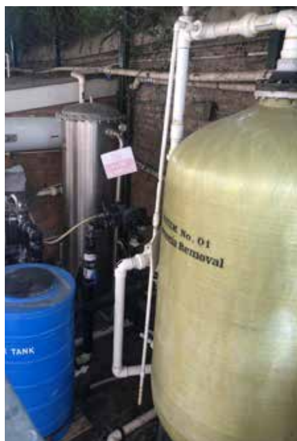
Final ammonia removal and polishing © Crown
