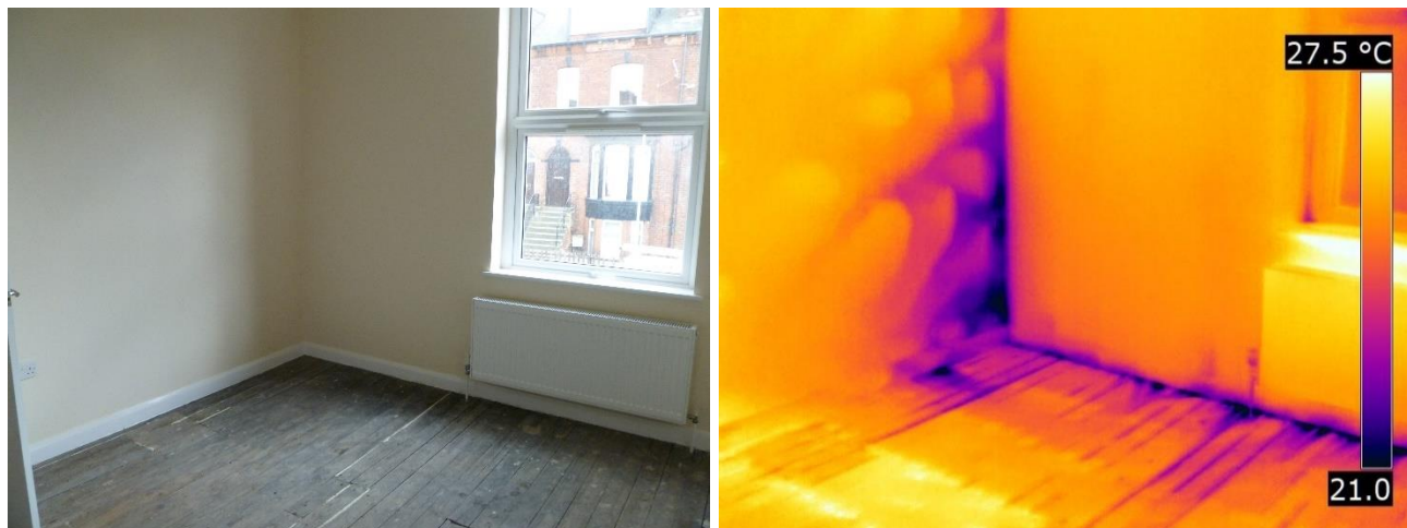
Figure 2-10 Thermal image taken under depressurisation illustrating a direct air leakage around the edges of internal wall insulation which is not adequately sealed [56]
