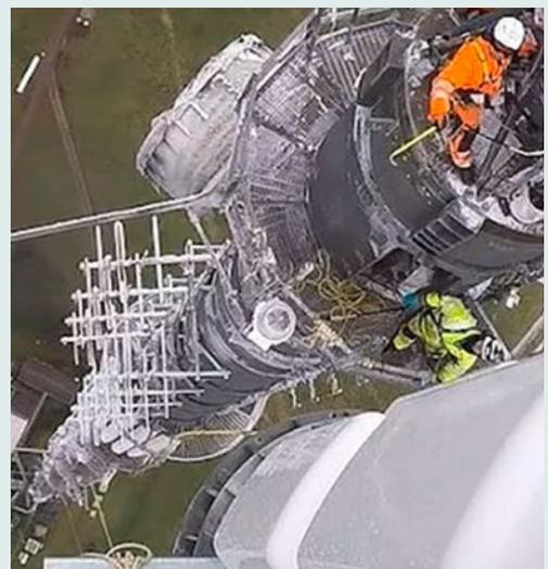
**A new antenna being lifted into place onto the top of a mast by a helicopter. Note the engineer waiting to "catch it".**
