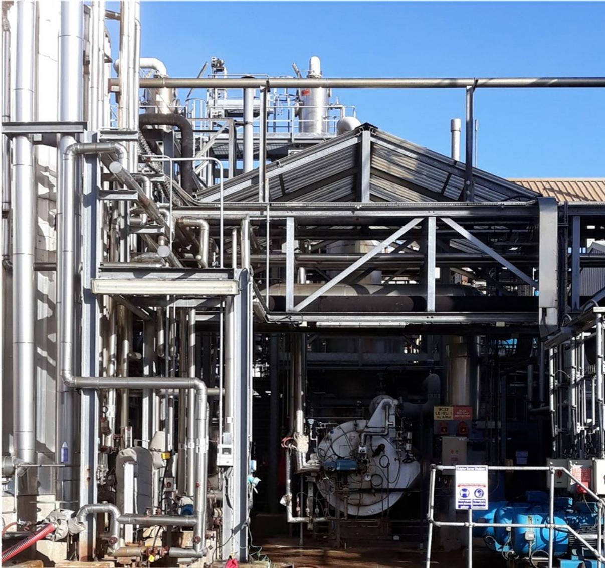
SULPHUR BURNER (FOREGROUND) Associated process plant & location for heat recovery to the rear.
