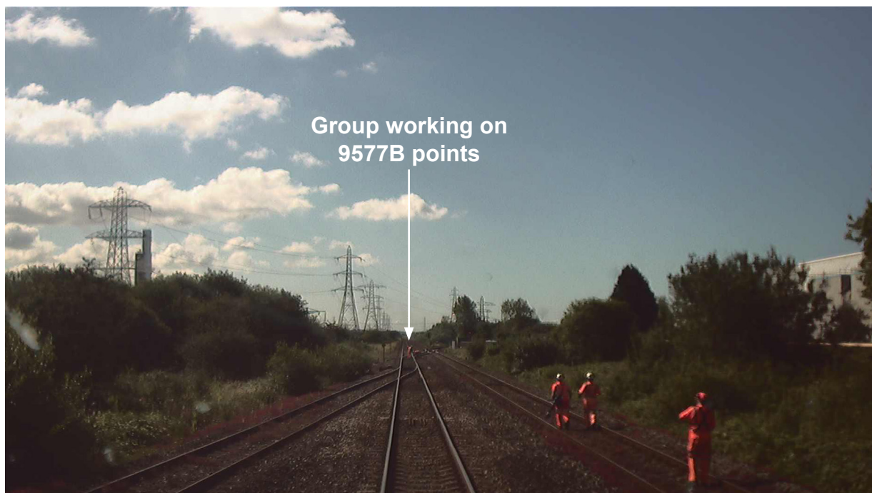
Figure 5: Image from forward-facing CCTV from train 1L48 as it was passing the group walking on the down main line
