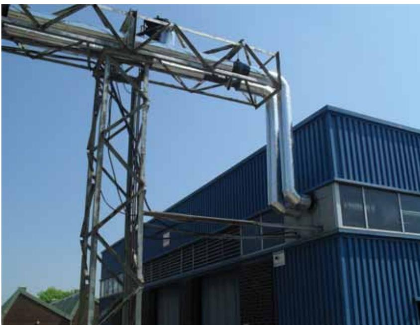
Replacement of insulation to the external high temperature hot water heating system at Boiler House 7, MOD Donnington © CarillionEnterprise
