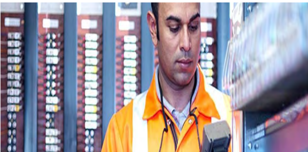
Engineer reading a meter in front of a wall of IT equipment.
