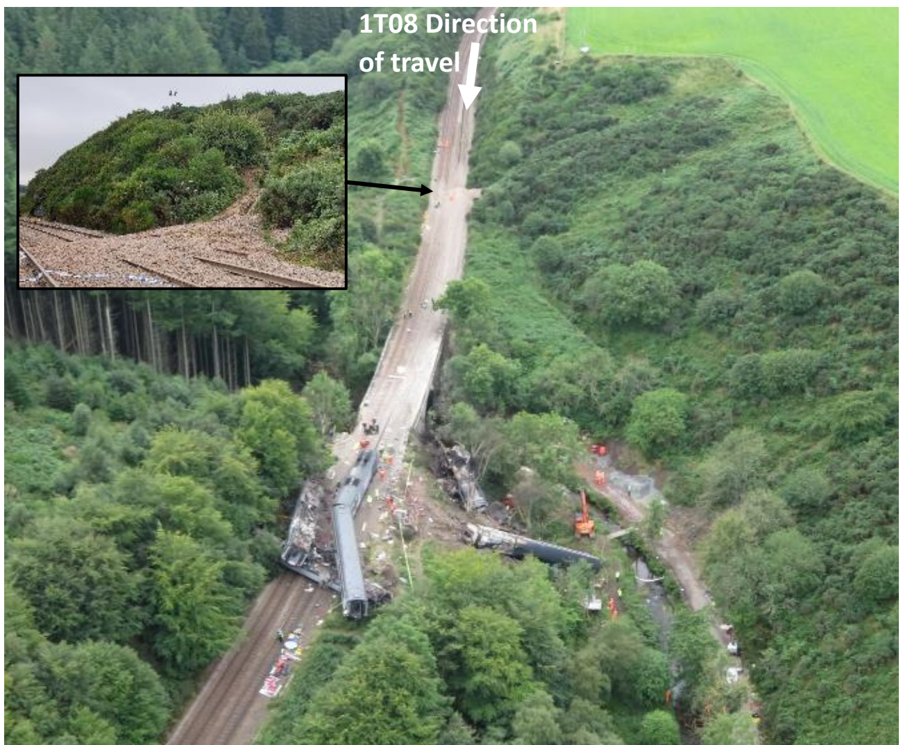
Figure 1. Aerial photograph of derailment site
