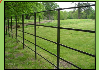
Estate railings to plots 6,7, 9 and 10
