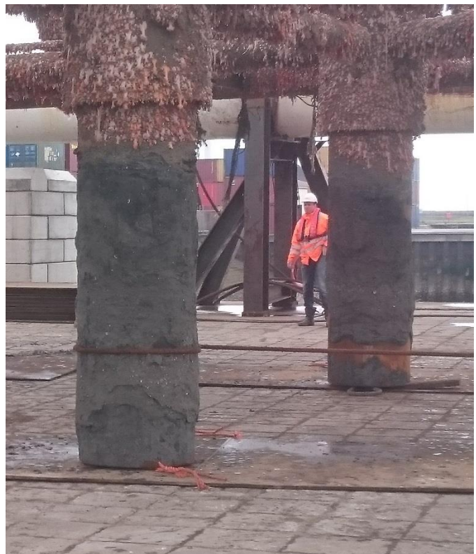
Fig 1.6 – Photos illustrating Stiff grey clay stuck to bottom 1.5 - 2.0m of cut WHPS pile
