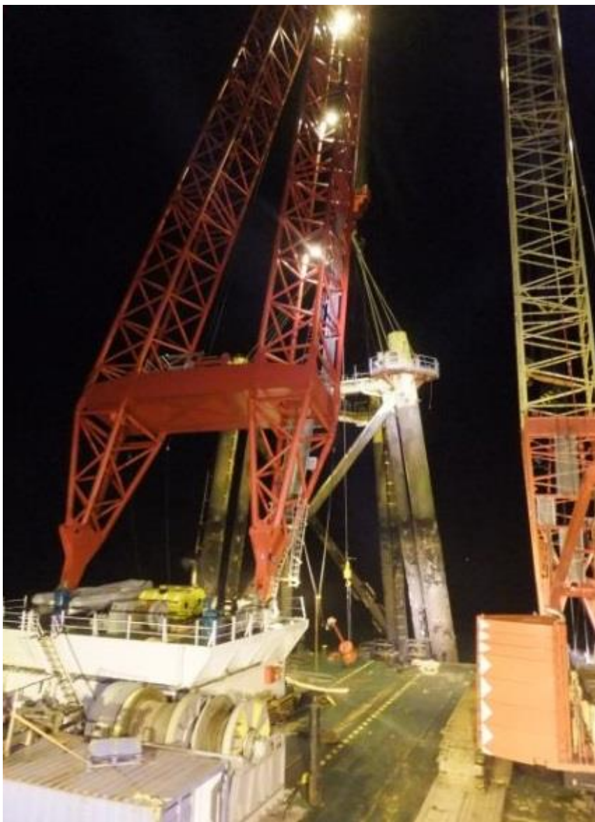
Fig 1.8 - Rambiz HLV Lifting Welland Jacket
