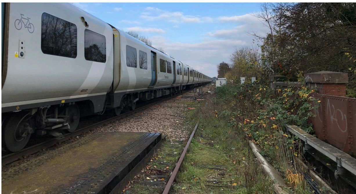
Figure 14: Image showing the down Redhill (slow) cess and walkway
