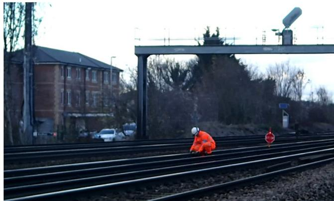
Figure 8: RAIB reconstruction showing protection (detonators and possession limit boards) being placed on up slow line
