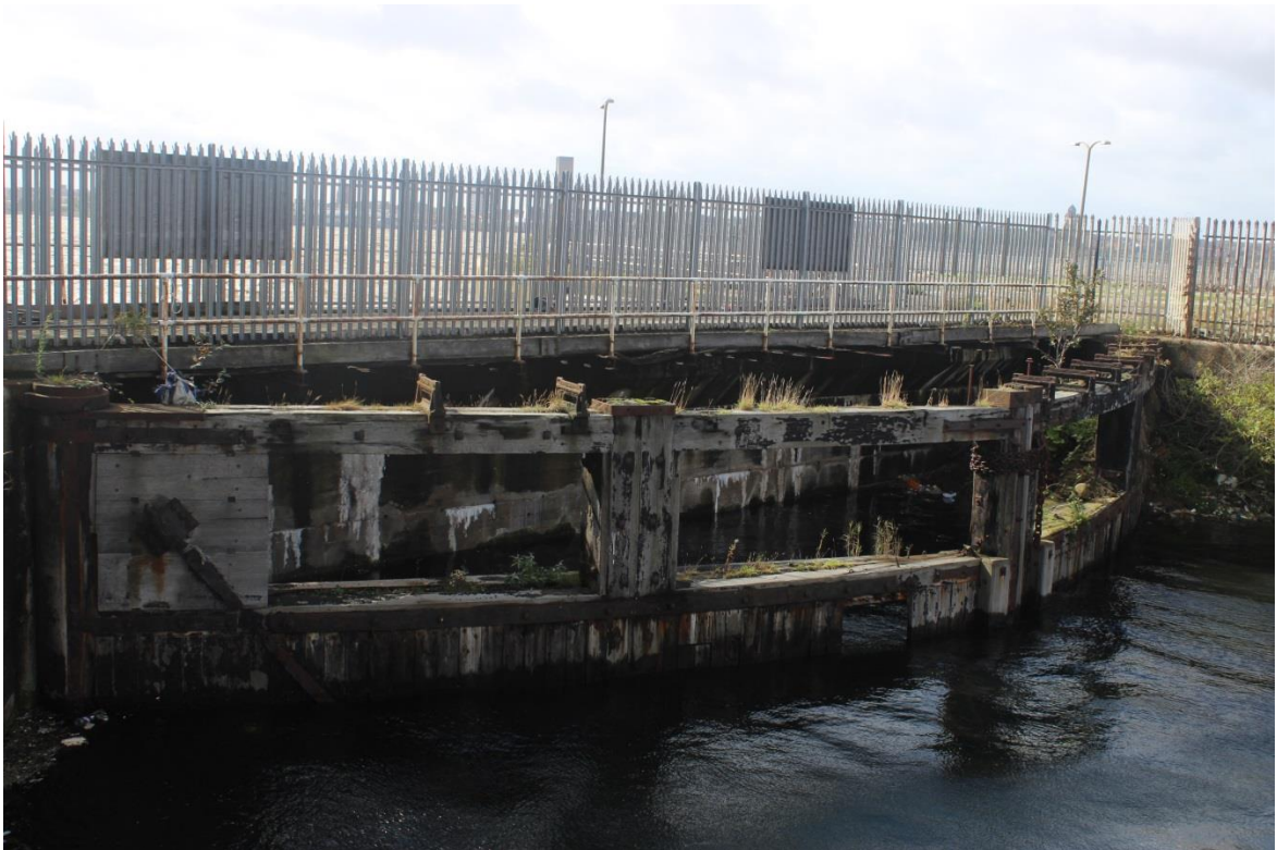
Figure 436: Princes Half Tide Dock Entrance
