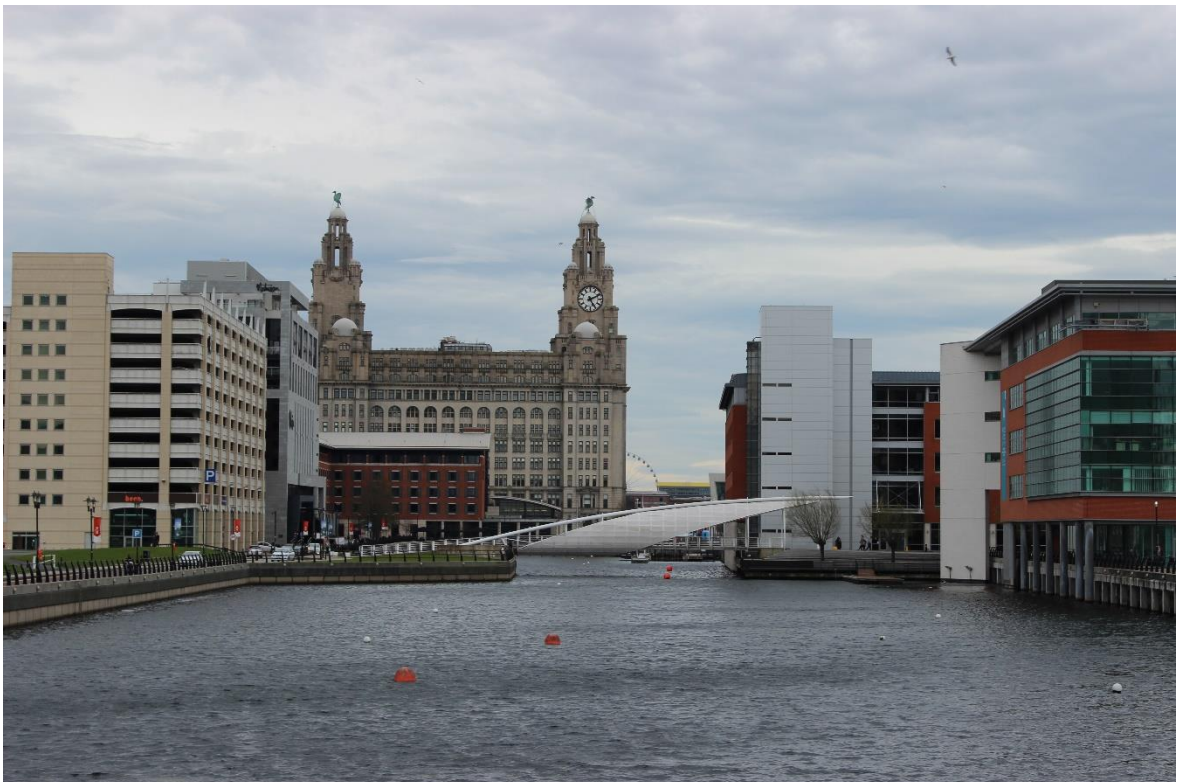
Figure 30: View South along Princes Dock towards the Royal Liver Building. The Site is on the right.
