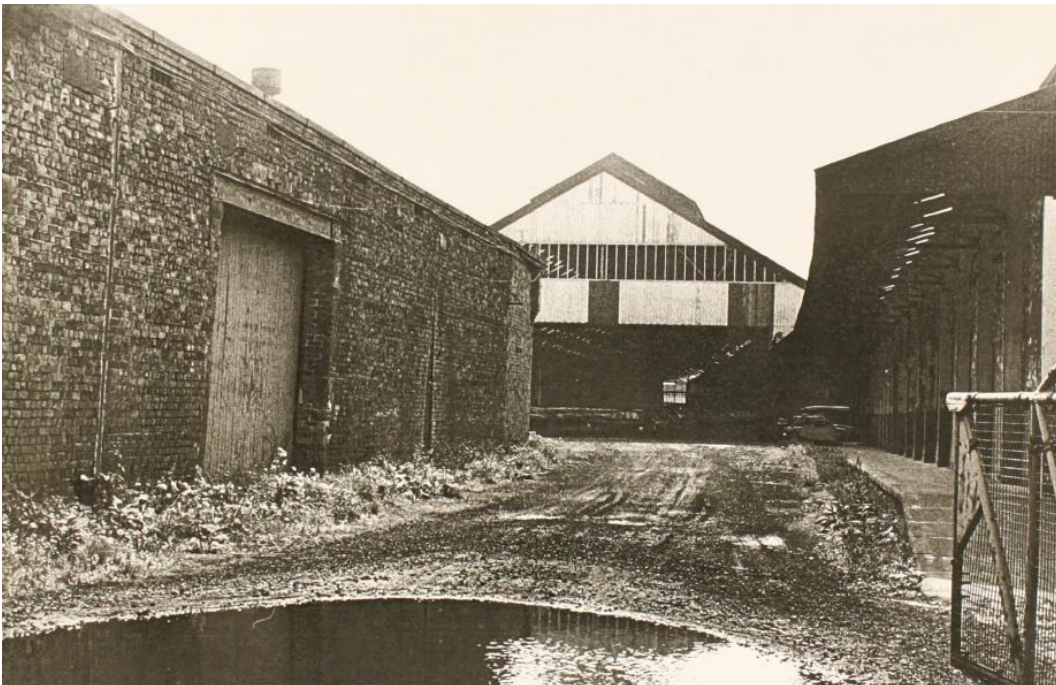
Figure 26: Entrance to Riverside Station, taken from within the area of the Site c.1981
