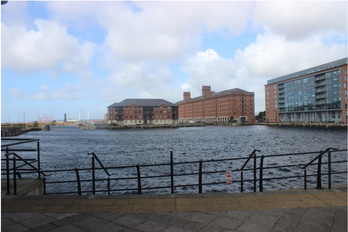
Figure 447: Princes Half Tide Dock with Waterloo Warehouse beyond (central building)
