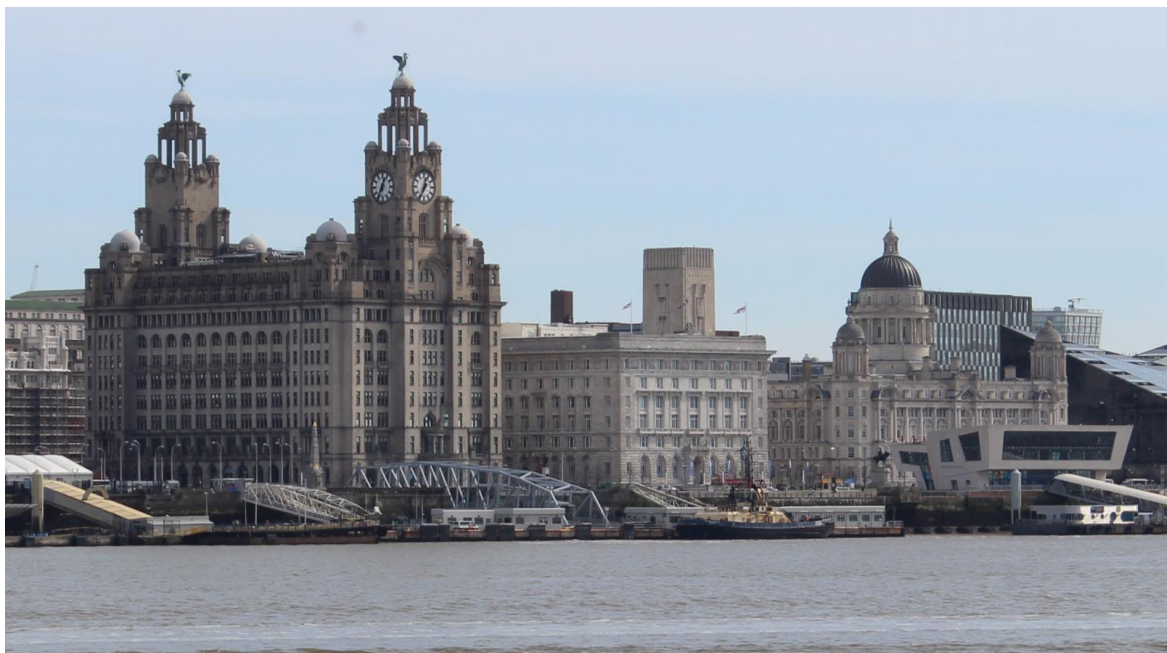
Figure 37: The Cunard Building in context with the other Three Graces
