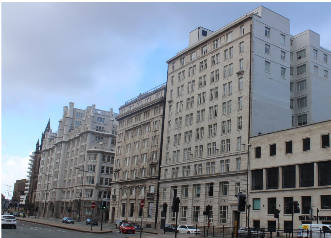
Figure 458: Wellington Buildings and West Africa House, with Tower Building beyond
