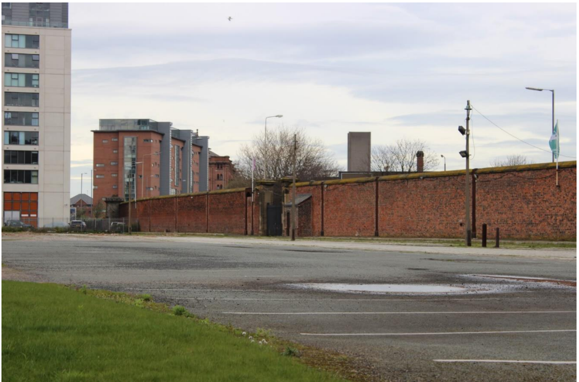
Figure 403: Princes Dock Wall and Gates
