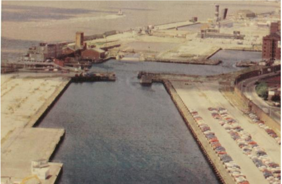
Figure 27: The cleared and derelict Princes Dock, c.1988
