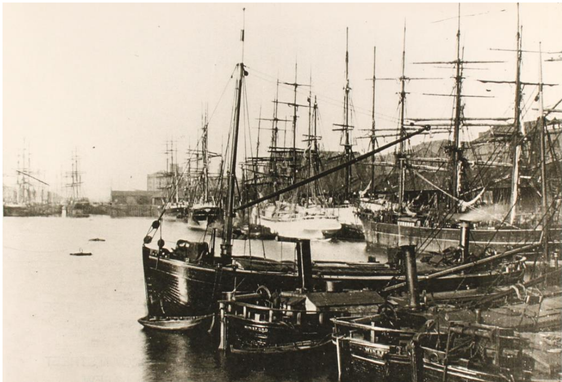
Figure 15: Photograph of Princes Dock looking north, c.1890. The Site would be on the left in this image.
