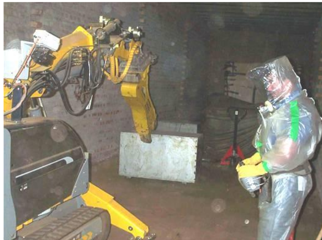
Figure 1: Air Fed Suit decommissioning work
