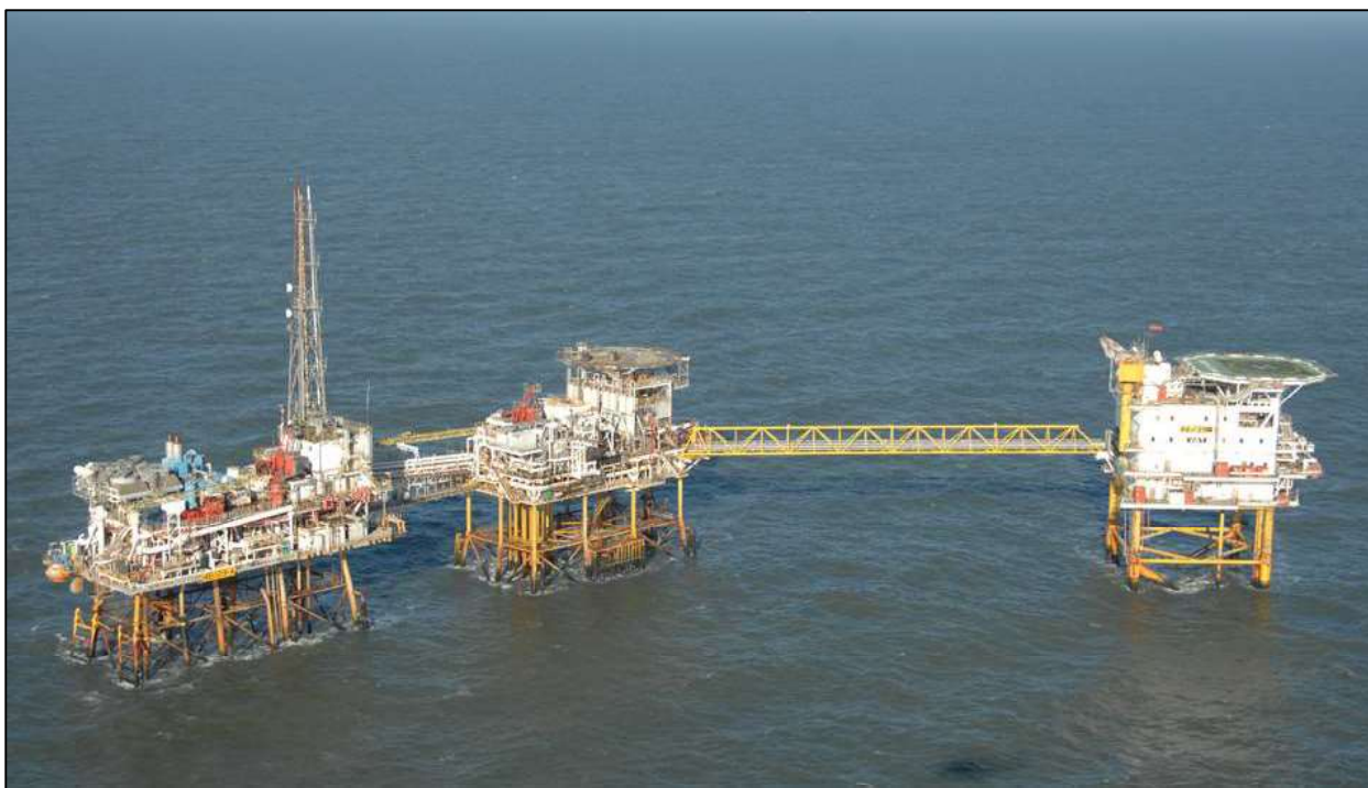
Figure 2.1 - Aerial View of 48/29A Complex
