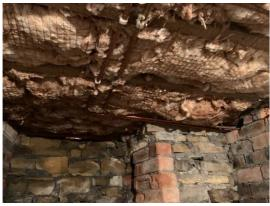
Image 6: Poorly secured insulation and covered electrical wiring
