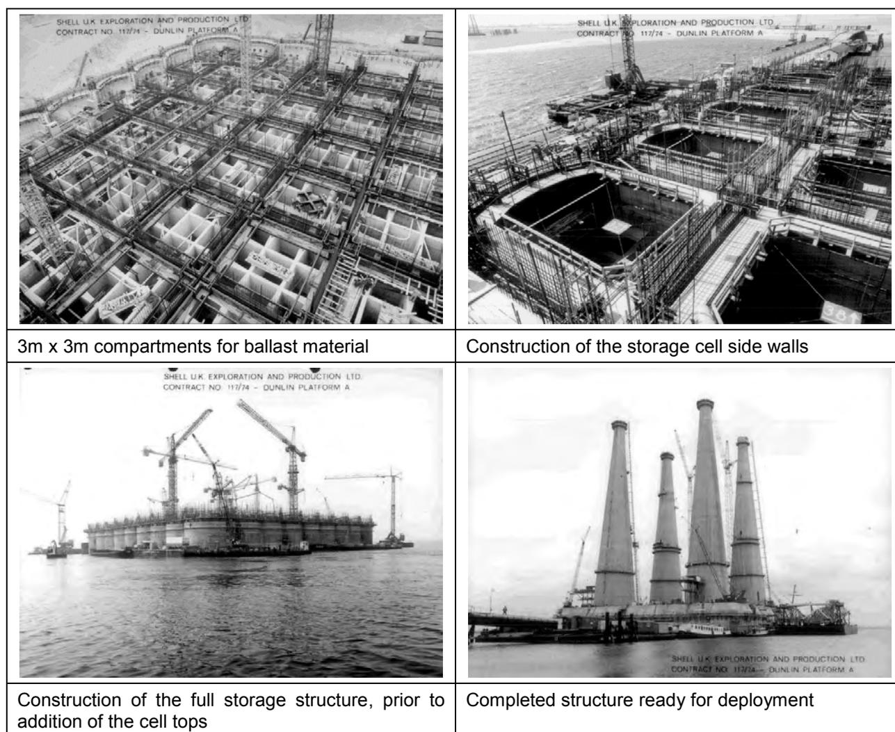
Figure 2.2 CGBS base and concrete legs during construction
