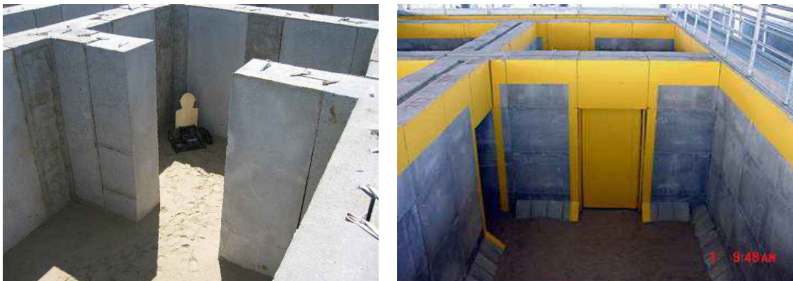
Fig 5 - 1. TARCON interlocking panels
