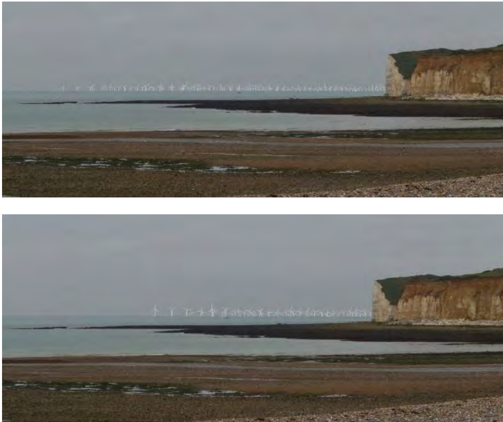
Top image: Option F with 175 3.6MW turbines. Bottom image: Option D with 100 7MW turbines
