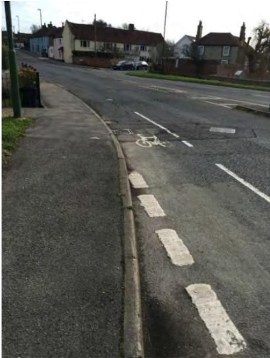
**Figure 3-8: Broken road surface with sunken drain covers**
