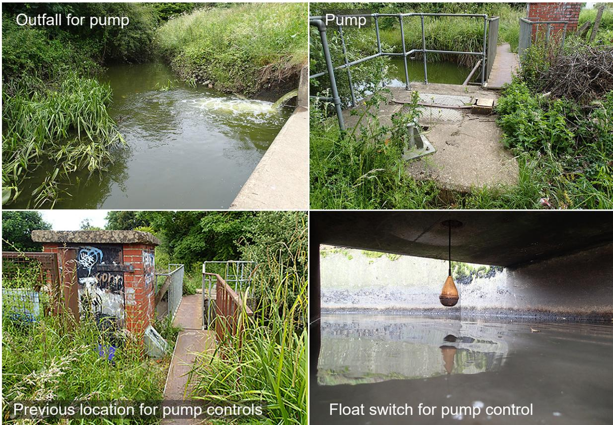
Figure 16: The pumping system at the spillways
