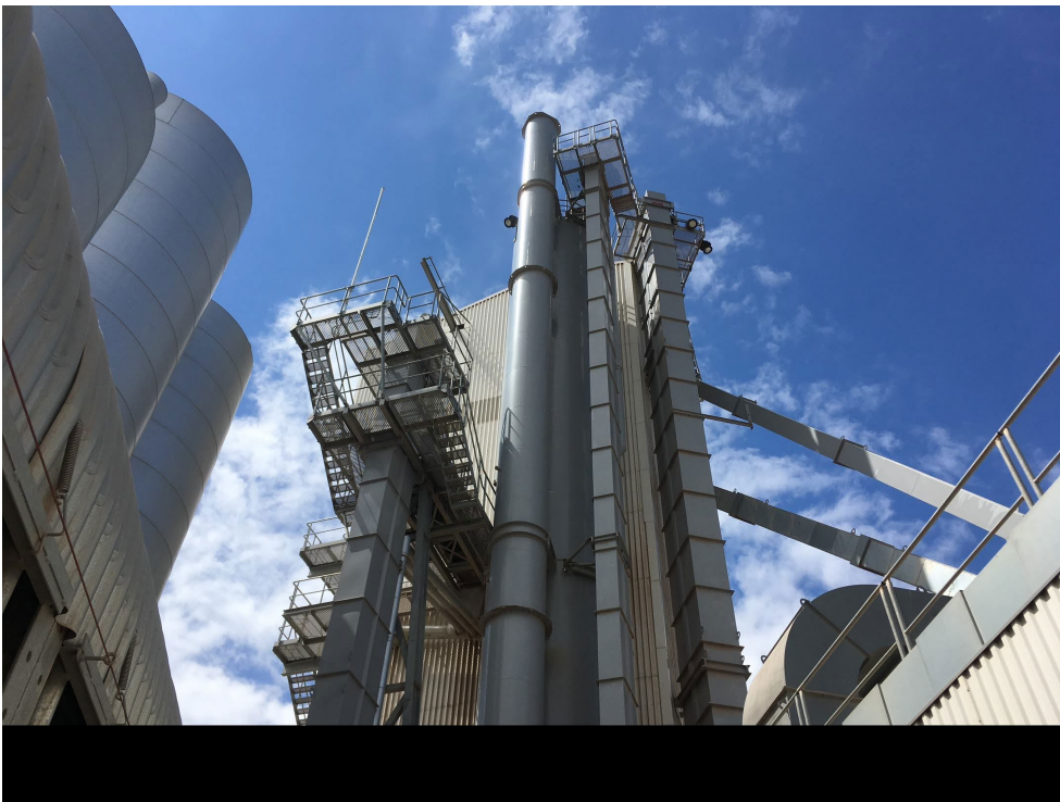
Avonmouth Asphalt Plant
