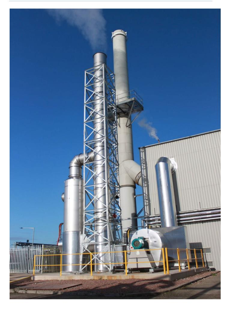
"The condensing economiser installation is the largest heat recovery project to be undertaken and successfully implemented at the Solutia UK Ltd Newport site. It will be partially funded by the IHRS programme and will serve to improve site energy efficiency and reduce our carbon footprint. The project has also helped raise site and employee awareness of the importance of energy efficiency, and has improved employee engagement in energy related matters"
