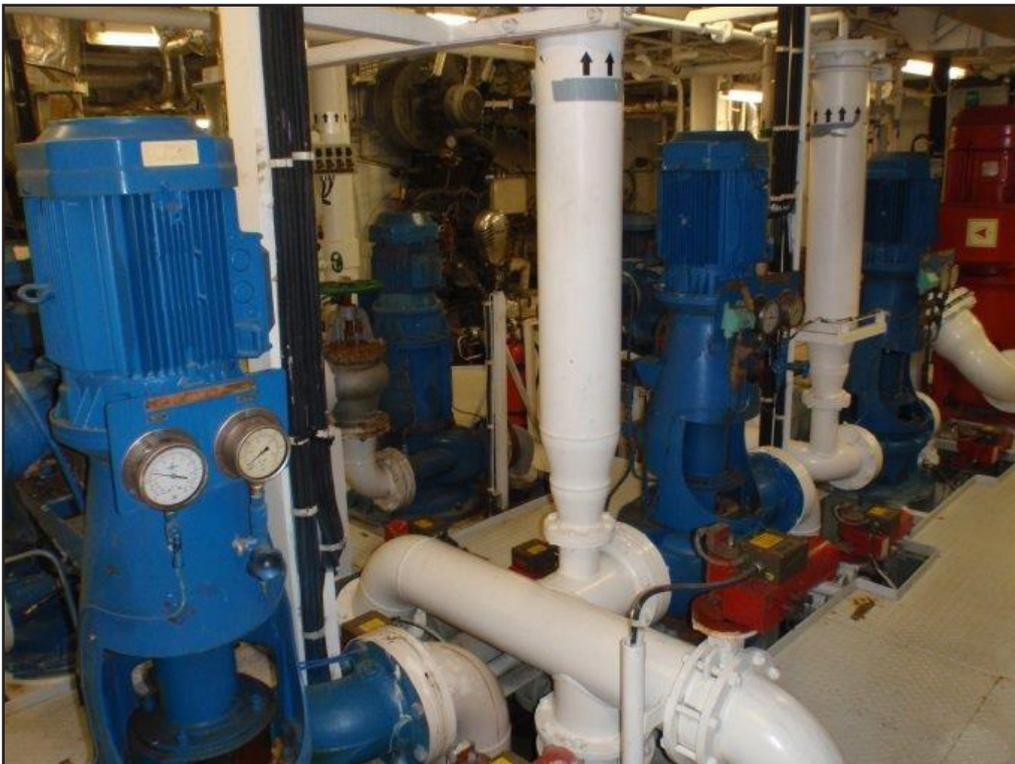
Figure 1: Bilge and ballast pumps and valves
