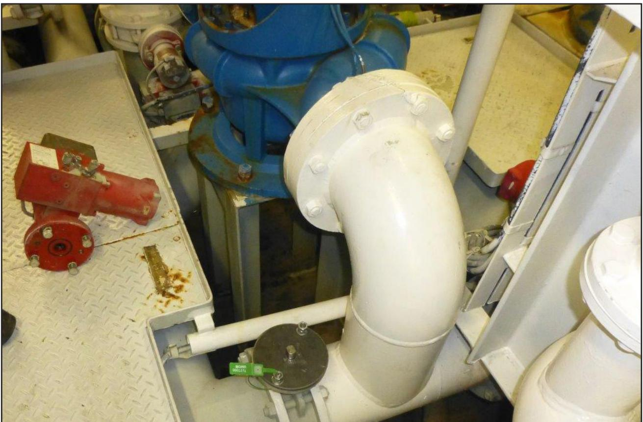
Figure 4: Modified cross-over valve - actuator removed, locking device fitted
