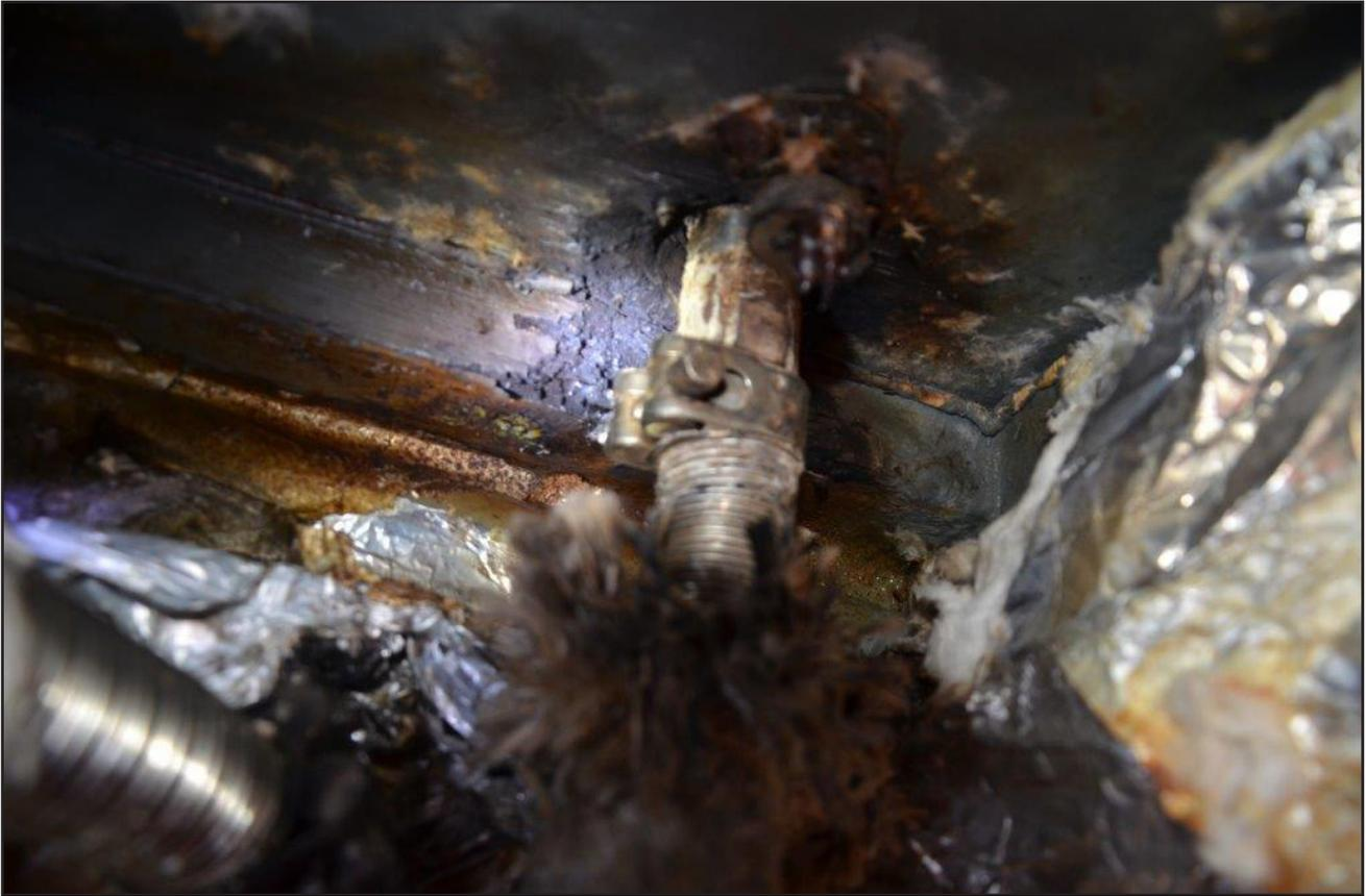
Figure 2: Uninsulated exhaust pipe causing the wooden deck to char
