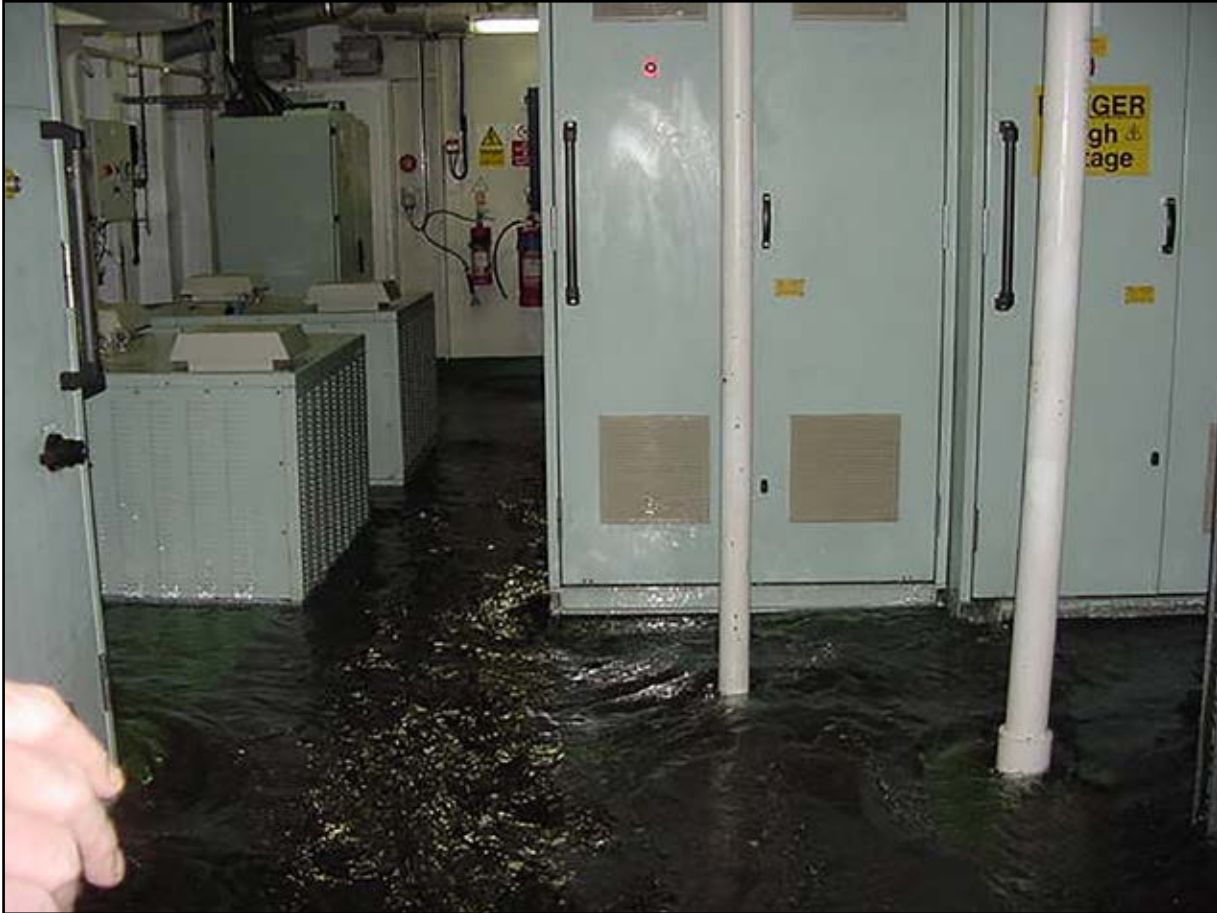
Figure 3: High voltage converter space
