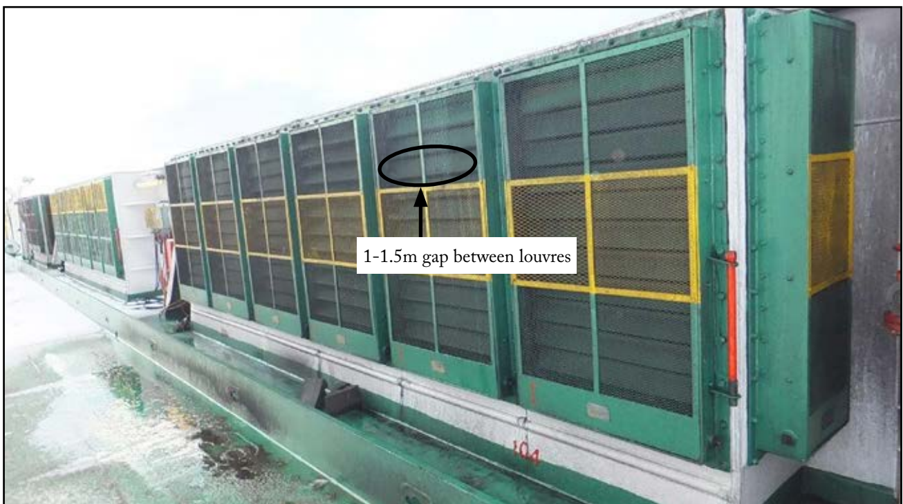
Figure 1: Ventilation jalousie and louvres arrangement
