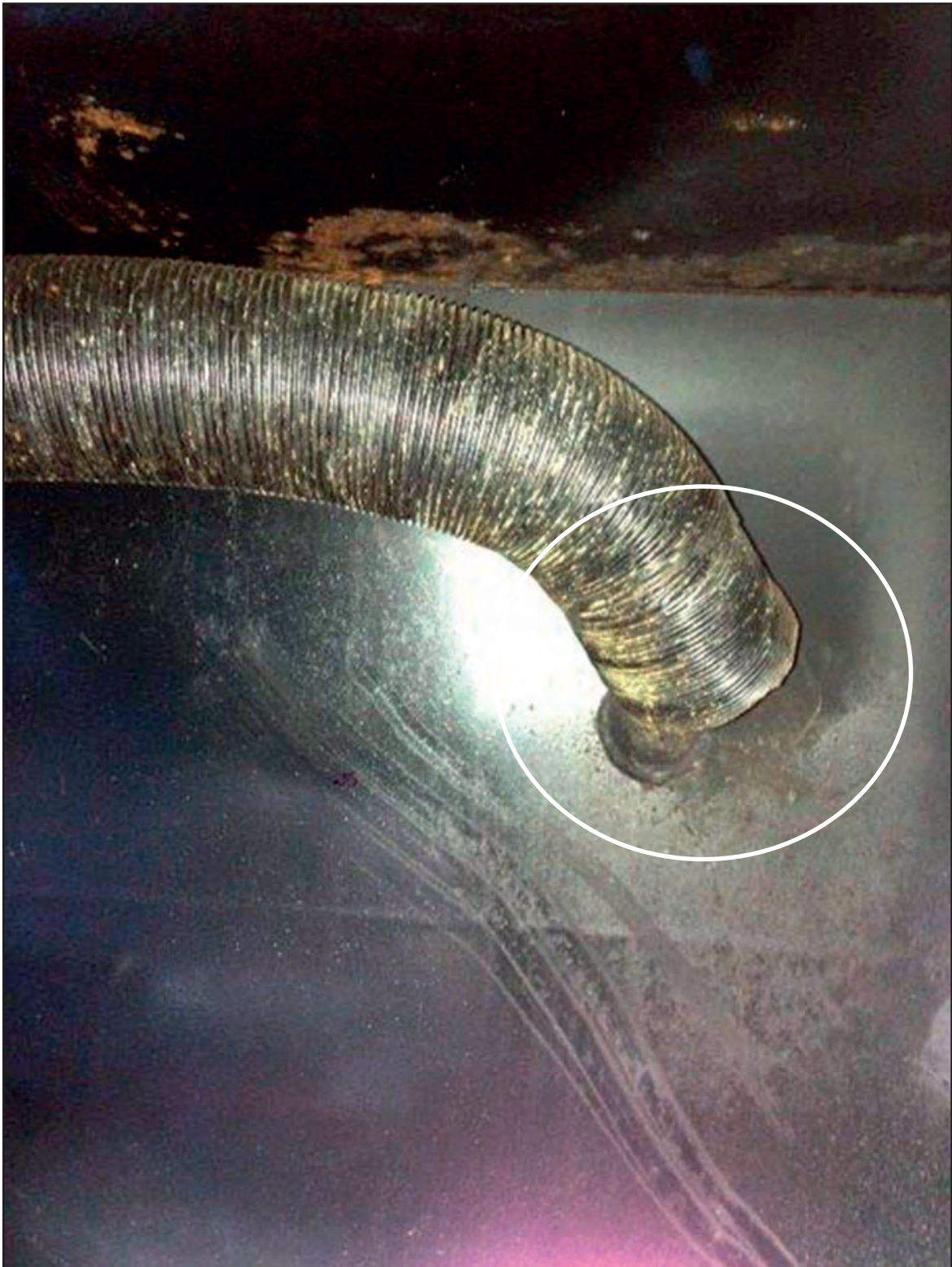
Figure 1: Soot staining around heater's exhaust
