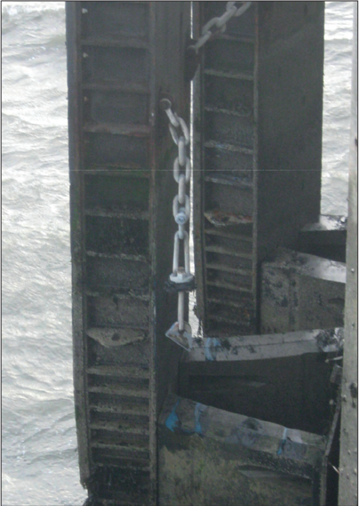
Figure 2: Damaged fender
