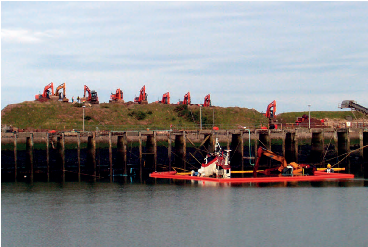
Excavators used to stabilise the dredger
