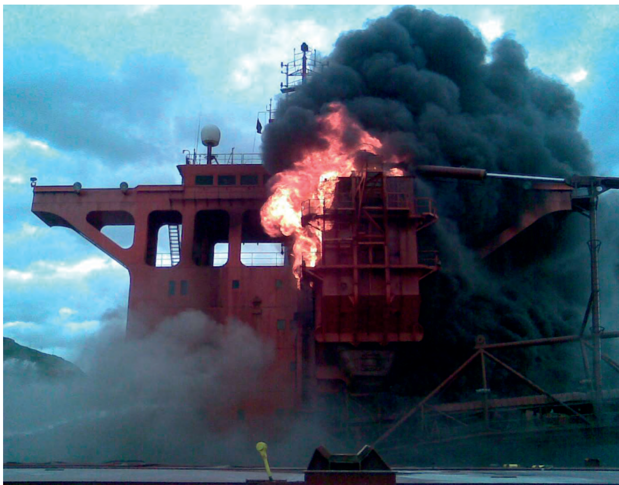
Figure 1: Fireball erupting from the vertical conveyor belt tower
