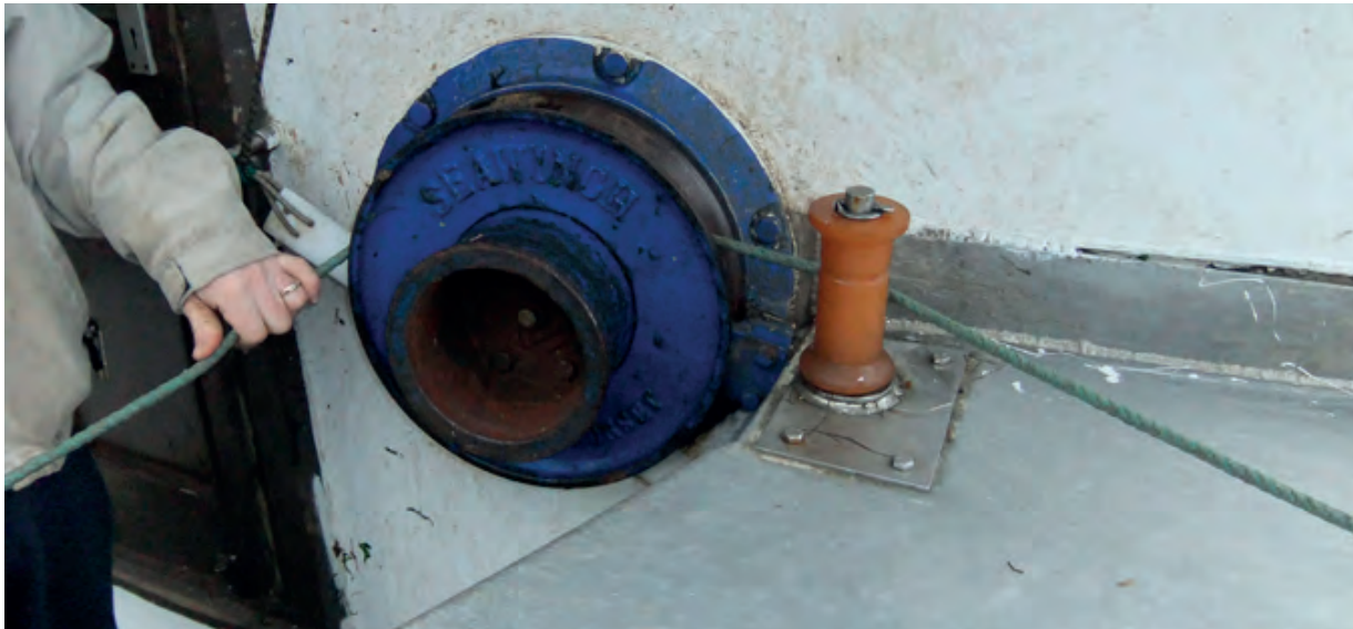
Figure 2: Additional vertical roller fitted close to the 'V' hauler
