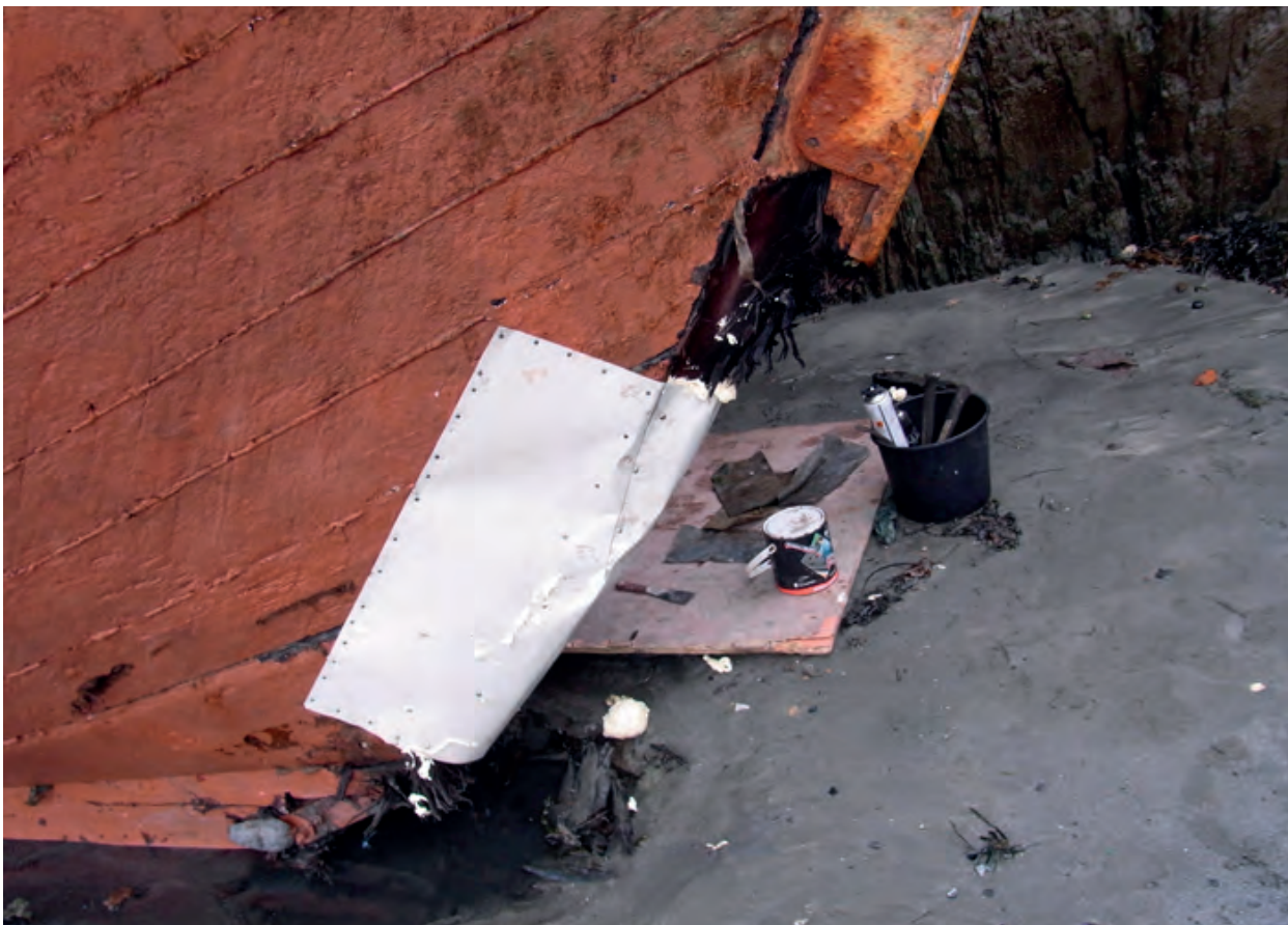
Figure 3: Stem post emergency repair
