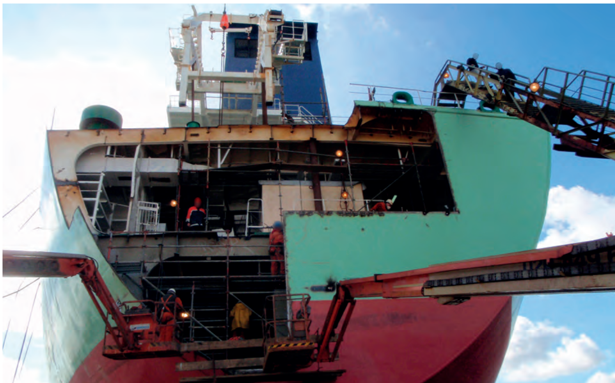
Repairs to the stern of the vessel discharging alongside
