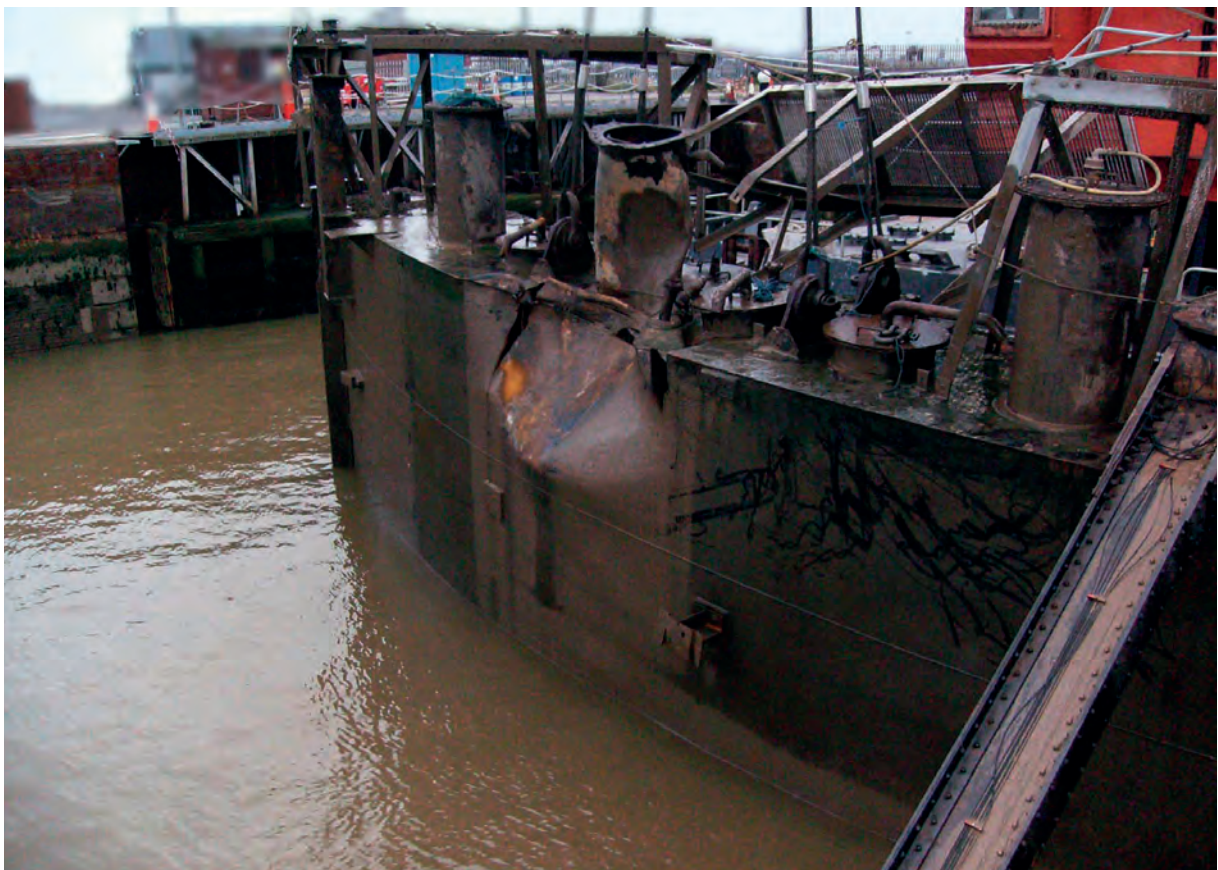
Figure 1: Salvage of sunken lock gate
