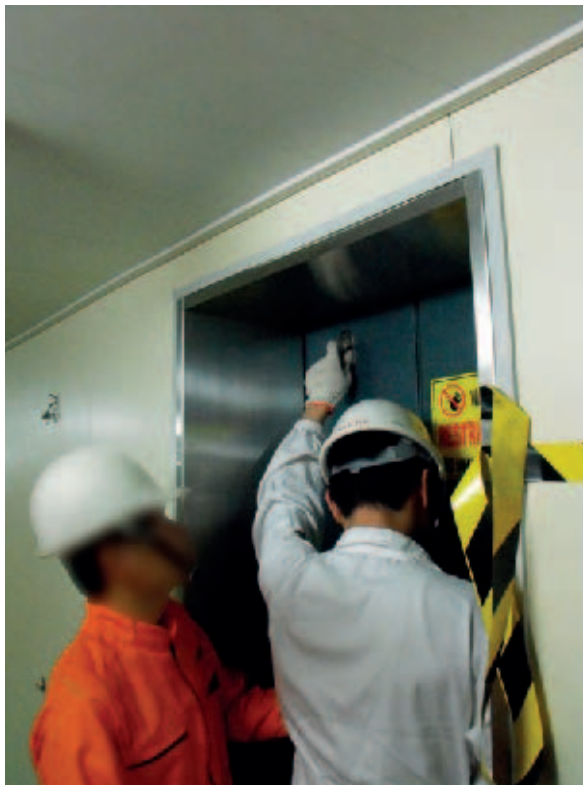
Figure 1: Lift shaft door being released
