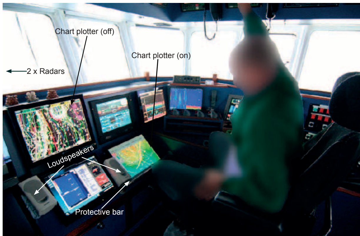
Figure 1: Wheelhouse looking forward to starboard
