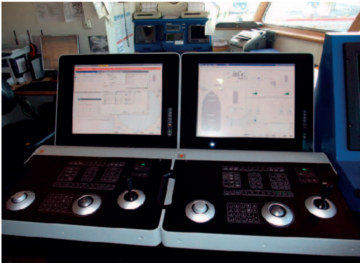
Figure 1: DP operator station
