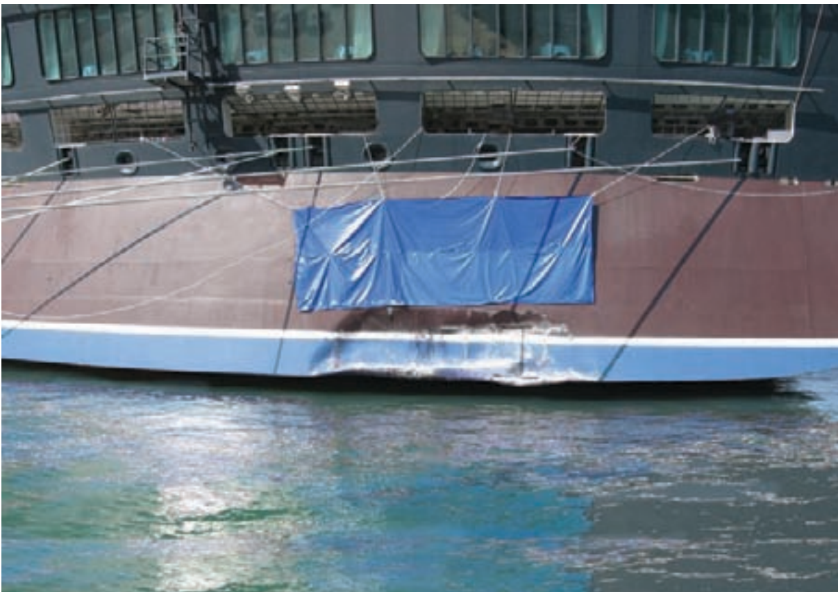
Figure 1: Damage to stern
