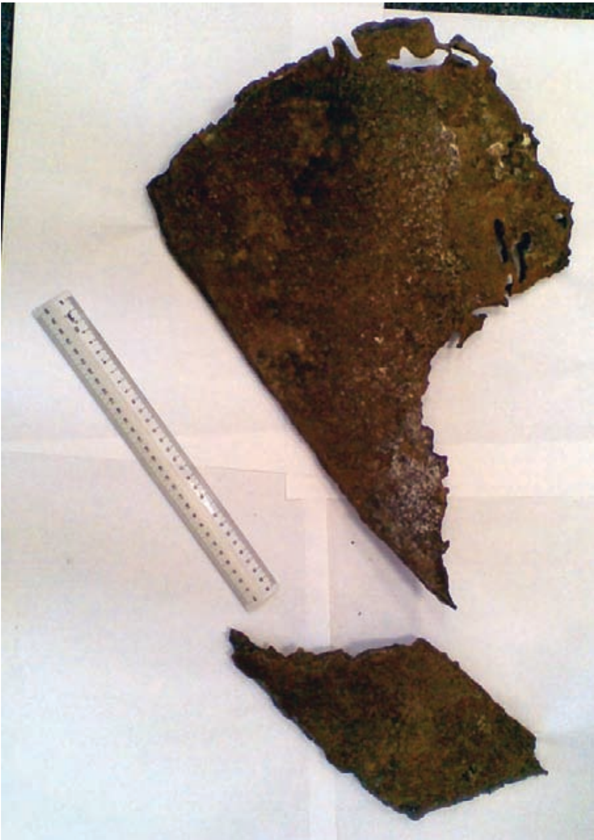
Figure 2: Removed steel protrusion
