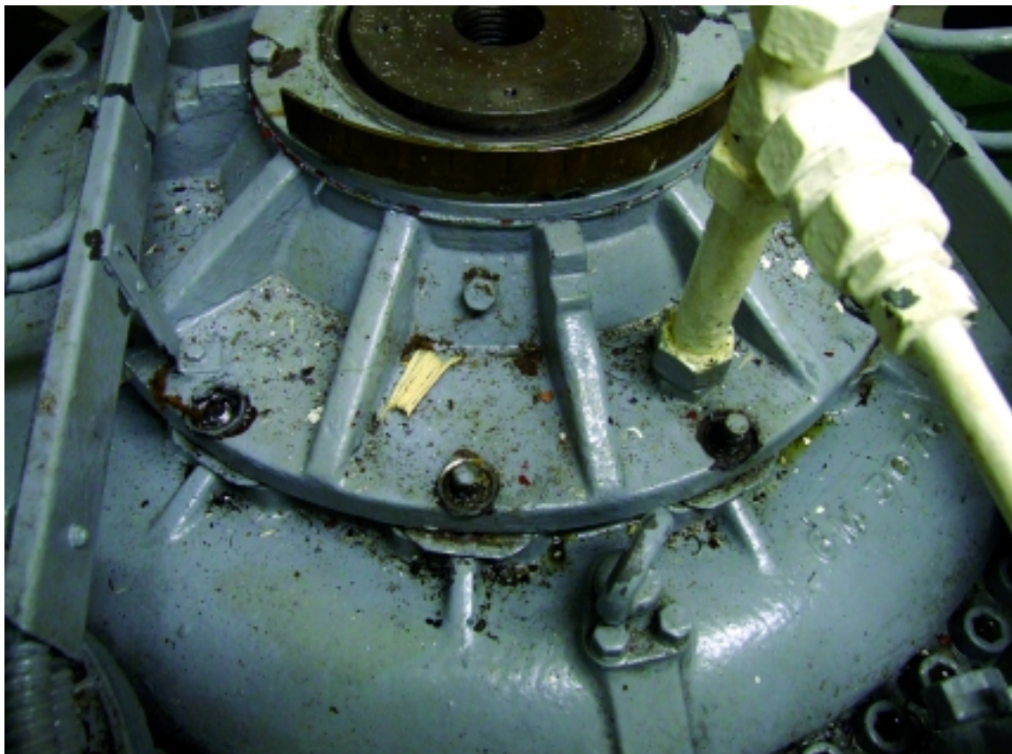
Figure 1: Damage to the vessel's steering gear
