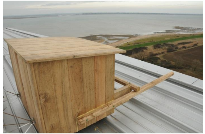
Figure 4: Fully mounted nesting box on the Reactor Building
