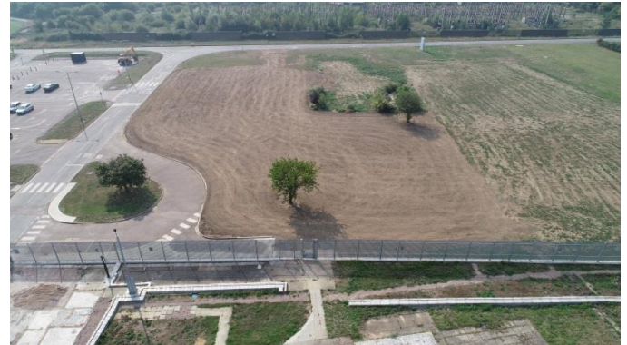
Figure 7: Remediation of the additional office and car park area used during C&MP
