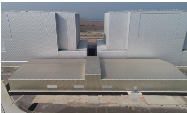
Figure 5: Image of the Ponds Building Complex Weather Envelope (foreground)
