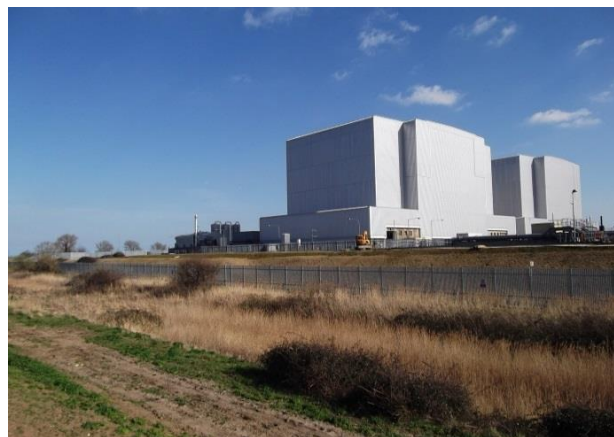
Figure 2: The Borrow Dyke
