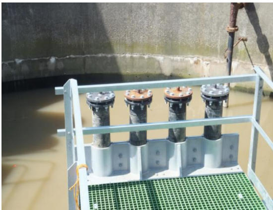
Figure 8: The four pipelines inside the East outlet culvert
