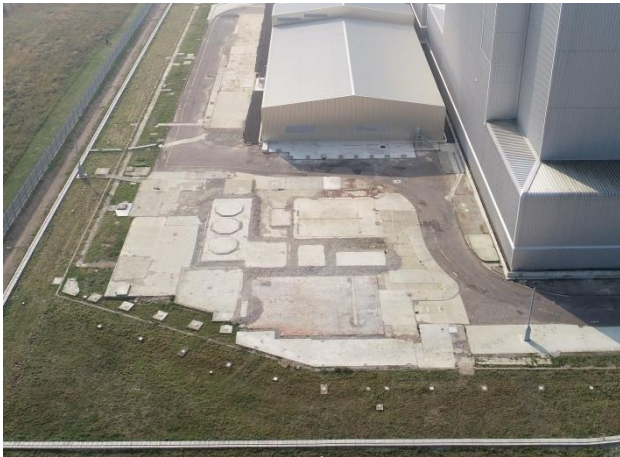
Figure 3: NO x Scrubber Tower area (now dismantled and demolished)
