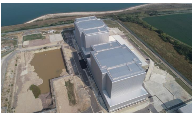
Figure 6: Image of the Reactor Safestore Weather Envelopes
